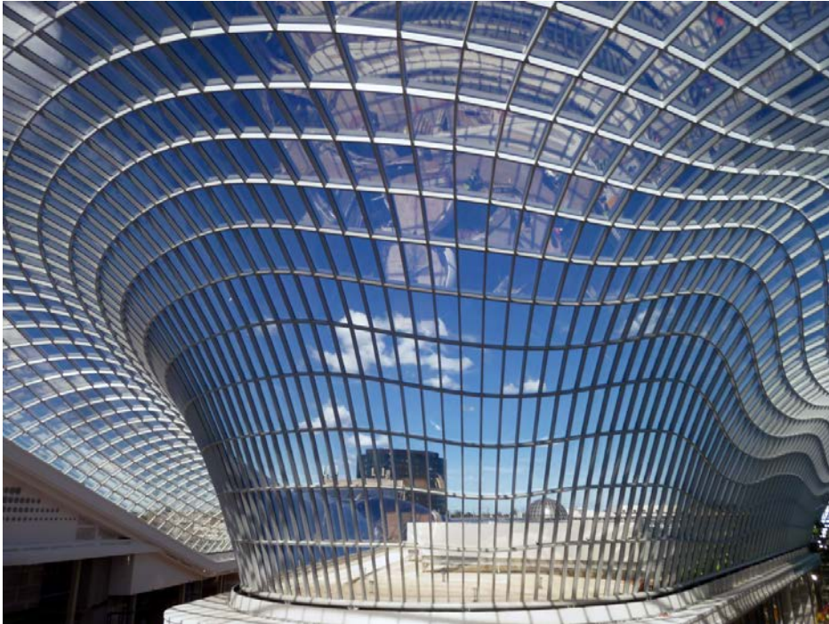
Chadstone Shopping Centre in Melbourne with spans of up to 44m. ©seele
