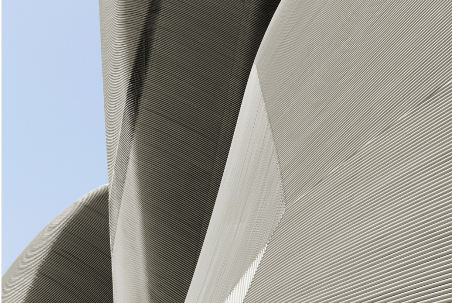
The façade wraps itself around the building without any steps. ©seele/Diemo Schillack
