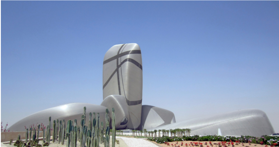
Situated in the heart of Saudi Arabia's oilfields, the King Abdulaziz Center for World Culture has a façade made from stainless steel tubes (total area: 30,260sqm). ©seele/Diemo Schillack
