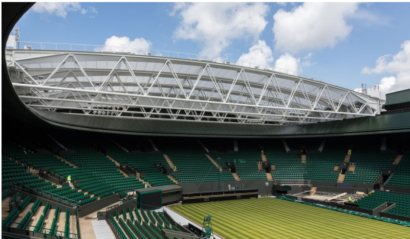
The 6,000sqm retractable membrane roof over Wimbledon's No.1 Court © seele
