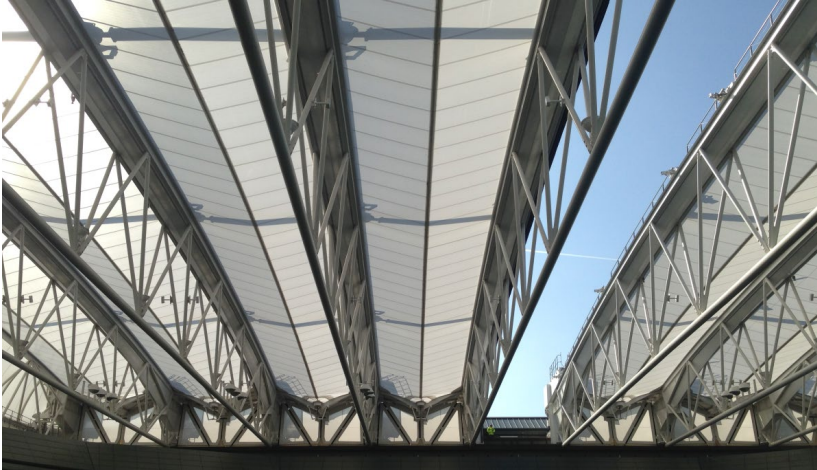
The membrane roof structure almost closed © seele
