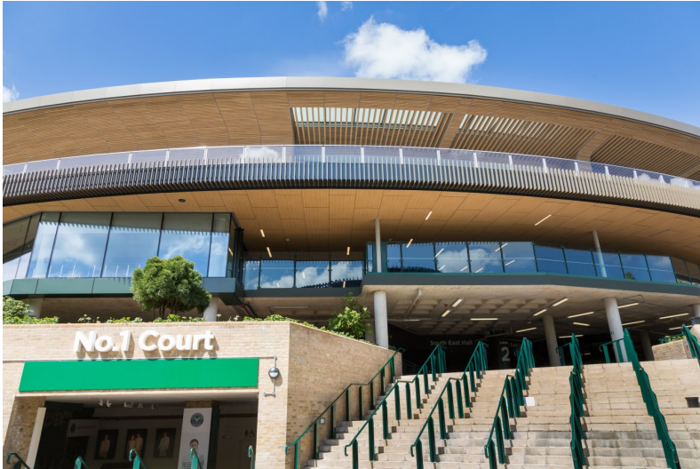
The fully refurbished No.1 Court at Wimbledon with its 13 different façade types and a retractable membrane roof by seele © seele
