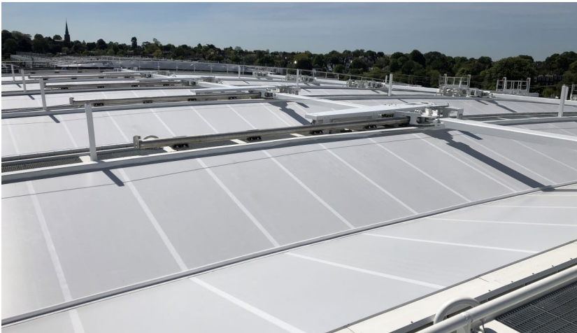
Each of the 10 membrane segments is made from 500sqm of PTFE material provided by seele © seele
