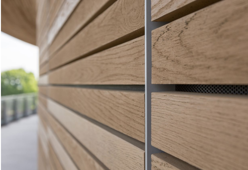
The panels are made from WPC slats attached to a perforated sheet metal supporting construction © seele
