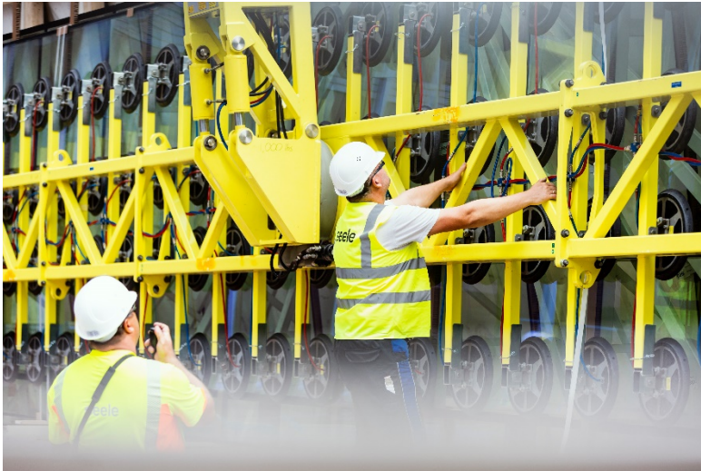
Special glass lifting apparatus with about 90 suction cups. © Jessica Schäfer
