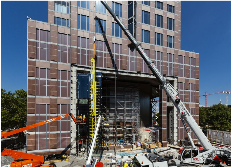
The first insulating glass units were set up in late July. © Jessica Schäfer
