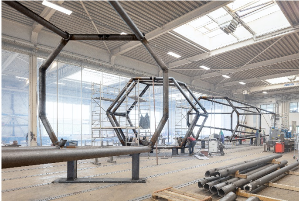
Steelwork fabrication in Plzeň © HG Esch
