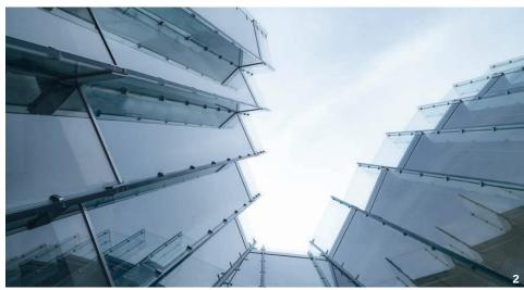
2 Glass fins form the supporting structure for the suspended all-glass construction. These were assembled from parts with lengths of up to either 16 m or 8 m.
