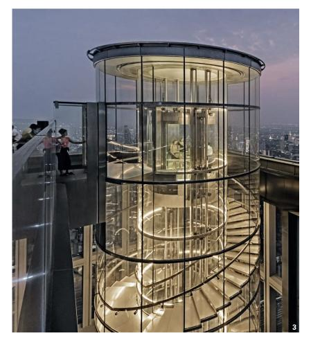
The 18 m high glass cylinder with its 600 sqm curved glass surface consists of an inner and an outer cylinder. Inside the cylinder a hydraulic lift extends over four floors. A spiral staircase was installed between the two glass cylinders. The peculiarity of the cylinder lies in the joints between the glasses: The prevailing weather conditions at the site required a system that provides the necessary stability of the entire cylinder.
