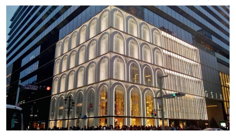
seele provided stainless steel arch elements with a special marble-look paint finish for the unconventional design by the architects from Curiosity. The 80 arch elements form 40 round arches that are screwed to the rectangular laminated glass panes via a supporting framework. Owing to the radius and their size, each deep-drawn stainless steel arch is made up of several separate parts that were welded together according to very tight tolerances so that the final appearance is impeccable.
