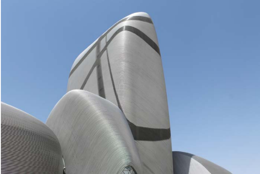
The façade of King Abdulaziz Center for World Culture consists of thousands of custom-formed stainless steel tubes. ©seele
