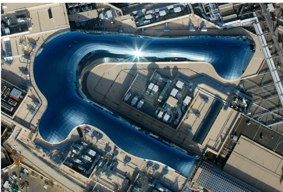
7080qm Freiform-Schalentragwerk Chadstone Shopping Center. ©seele
