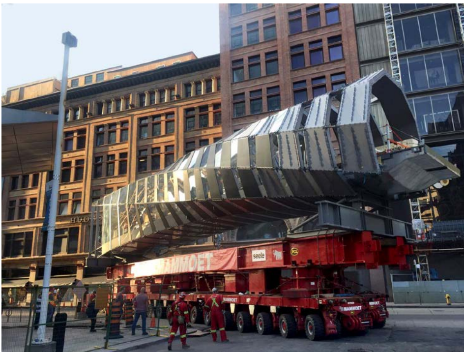
Transport of the new CF TEC Bridge to its final position. ©seele
