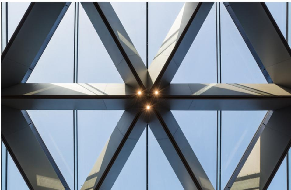
The multi-function roof structure with its mainly triangular panes of insulating glass ©James Newton
