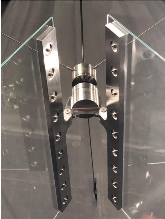
Two sheets of thin glass elegantly bonded to stainless-steel edge strips are suspended from a tripod structure which holds the swinging car very close over a podium.
