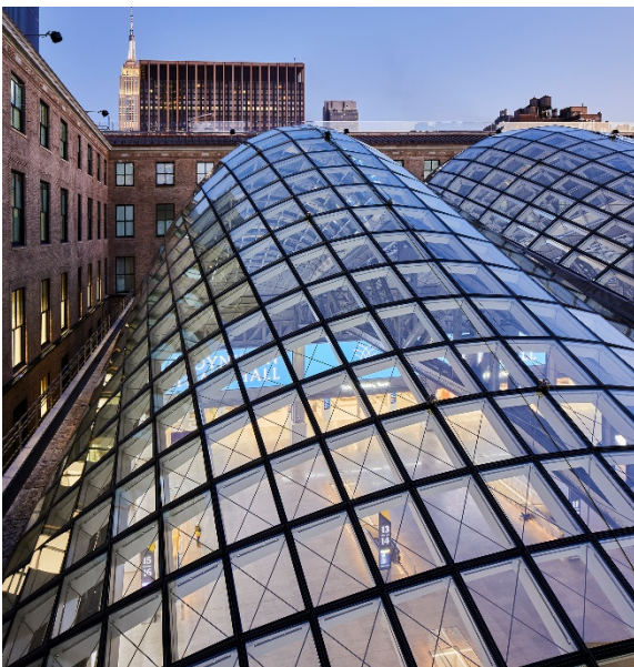
seele was also responsible for approx. 5,000 sqm roof constructions at Moynihan Train Hall, New York, which opened on January, 2021.
