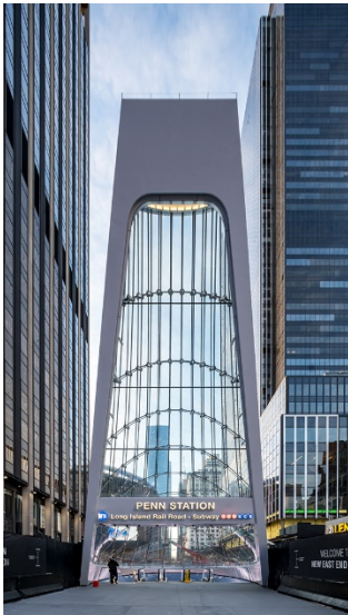
A 12m high, inclined "A" forms the new entrance to Penn Station, New York's largest railway station. © Field Condition
