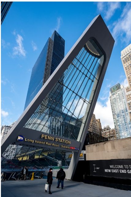
The new entrance to Penn Station on 33rd Street consists of a steel frame at an angle of 45° and a double-curvature cable net façade. © Field Condition
