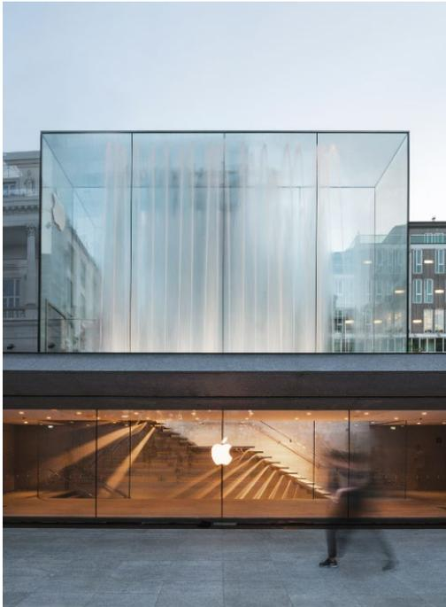
Entrance to Apple Retail Store in Milan, the two long sides of which consist of just four panes each. The special feature here is that the glass is not connected by stainless steel fixings, instead merely by silicone adhesive joints. © Giovanni Nardi Photography
